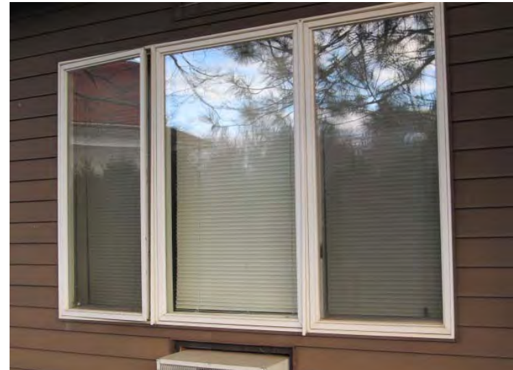
Original windows are in generally good condition for their age – No operational problems noted
