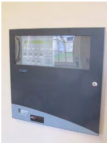
Fully addressable fire alarm control panel – Entire system was upgraded in 2009
