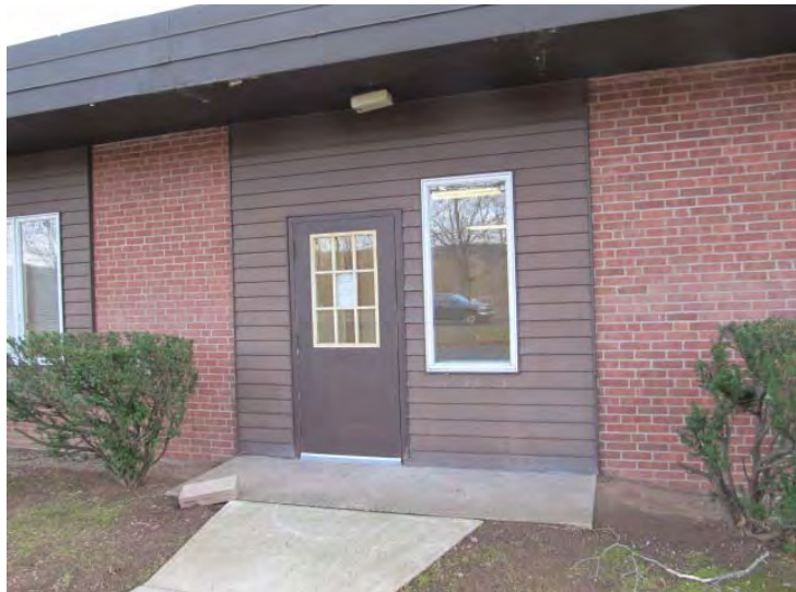
Exterior wall surfaces are a mix of (exposed and painted masonry) and aluminum siding
