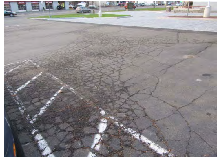
Asphalt-paved parking areas exhibit cracks and wear
