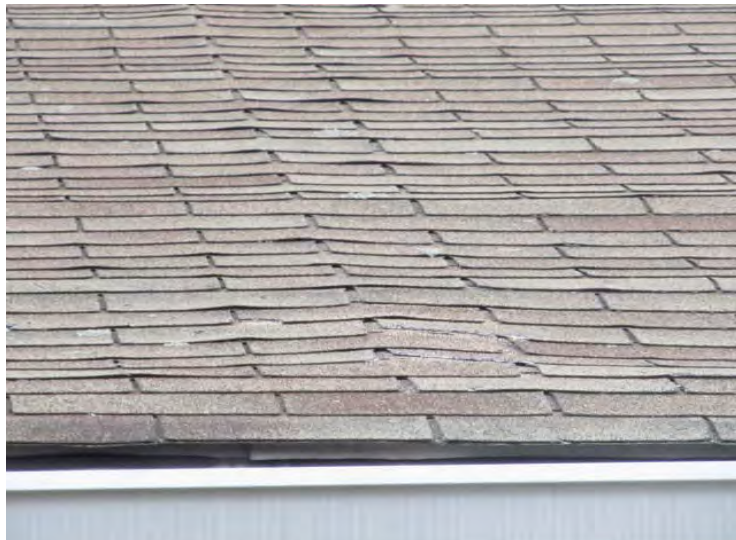
Roof shingles at pitched roof area are original and exhibit signs of age-related wear
