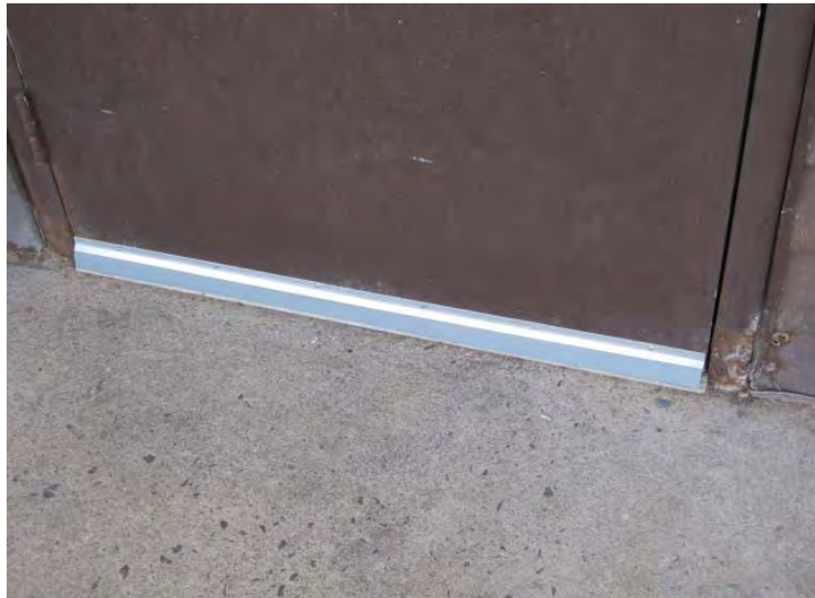
Rust-damaged frame noted at secondary building entry door
