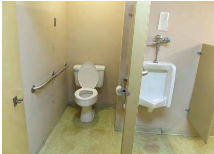
Vinyl sheet floor coverings in restrooms are in need of replacement in the near-term
