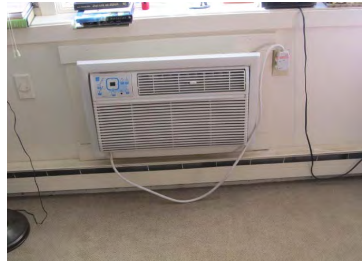
Each unit is provided with a thru-wall air conditioner for space cooling needs
