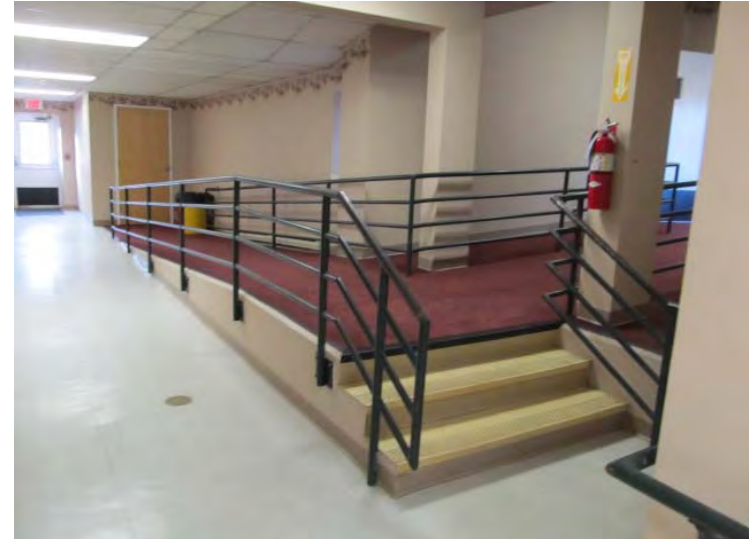
Portion of ramp system for handicap access between southwest and northwest sections of building
