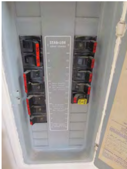
Typical 'Stab-Lok' circuit breaker panel found in each unit – Panels of this type and brand have a history of failure and service parts are unavailable
