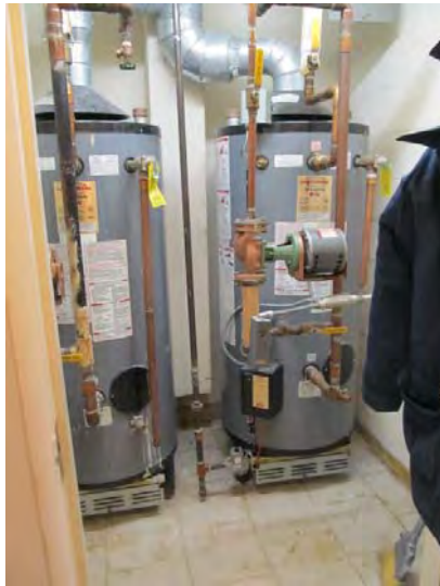
Two of three commercial-type gas-fired domestic hot water tanks that serve the residential units
