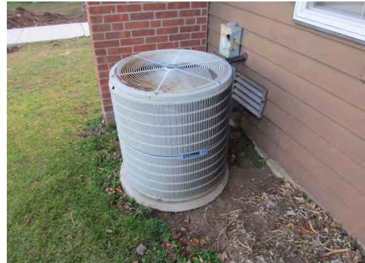
Older, exterior-mounted, condenser for cooling of selective interior common areas
